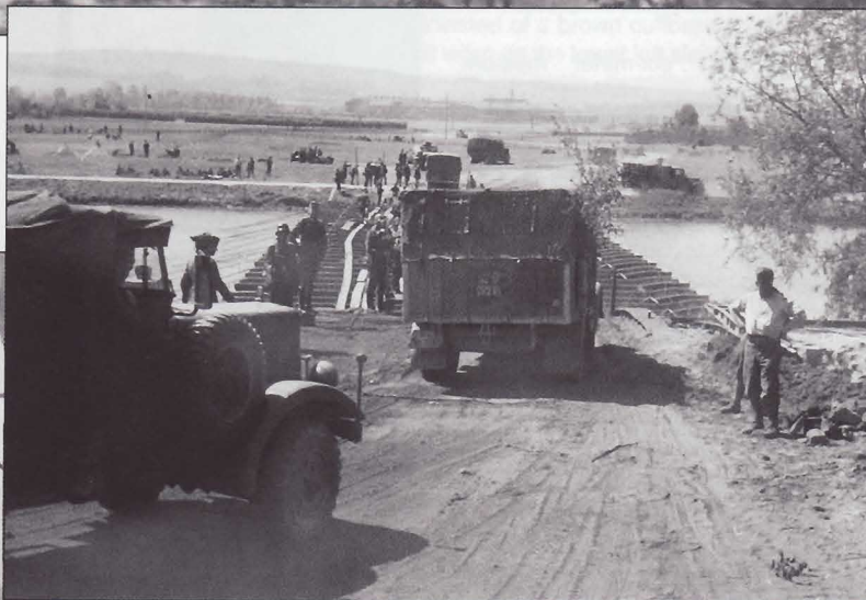
A combination fixed-type and pontoon bridge. This combination was employed when the bottom was too shallow to float pontoon boats. It is difficult to identify specific types of trucks as there were so many different makes and models employed to include commercial models and vehicles commandeered or purchased before the war from Czechoslovakia, Austria, Poland, etc. Truck "45" passing through this burning town was built by Ford Werke of Cologne.
