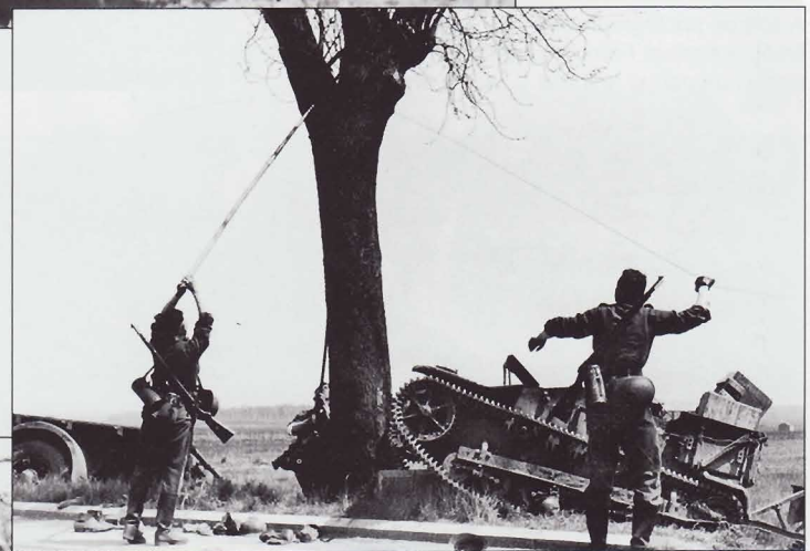
Signals troops string a field telephone line with the aid of a lineman's pole to bridge a road. Friendly vehicle traffic caused more telephone line breaks than enemy fire. On the roadside sits a French Chenillette Mle 1931R tractor and its little full-tracked limber (mostly unseen in the ditch) used to tow 25mm Mle 1934 and Mle 1937 antitank guns, which proved to be totally inadequate weapons even in 1940.
