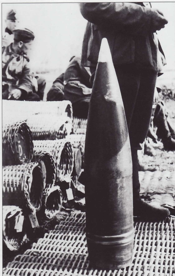
A 95.7-pound (44.226-kilogram) 15cm high-explosive projectile. The 15cm sFH 18 heavy field howitzer was also provided armor-piercing, anti-concrete, and smoke projectiles. The projectiles were shipped in wicker containers.
