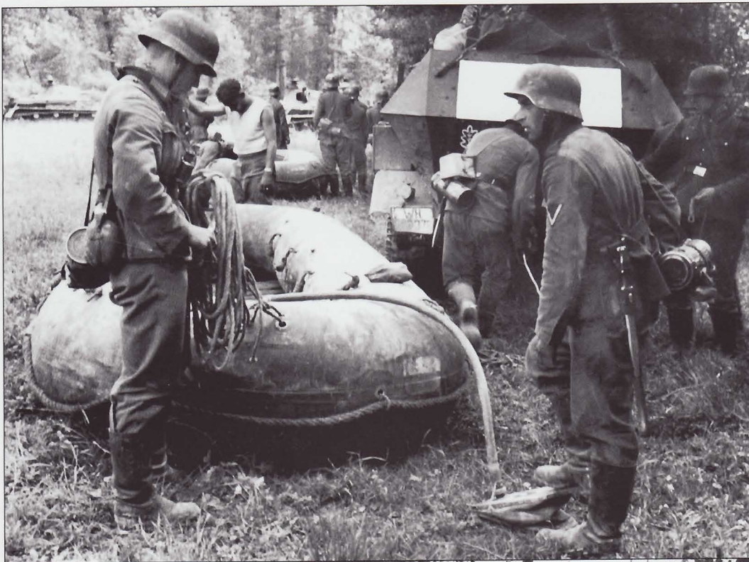
Soldiers inflate six-meter medium pneumatic boats in preparation for a stream crossing. Note the foot-operated inflation pump. In the background is an SdKfz 250/1 halftrack. Note the white or yellow panel painted on its rear. This served as air-to-ground recognition. Often orange fabric panels were used for this purpose. Partly obscured is the white oak leaf insignia of 1. Panzer-Division. Inflated the boat weighed 330 pounds (150 kilograms). Here, because of the stream's swift current and narrow width a simple hand-over-hand line has been installed for boat crews to pull themselves across.
