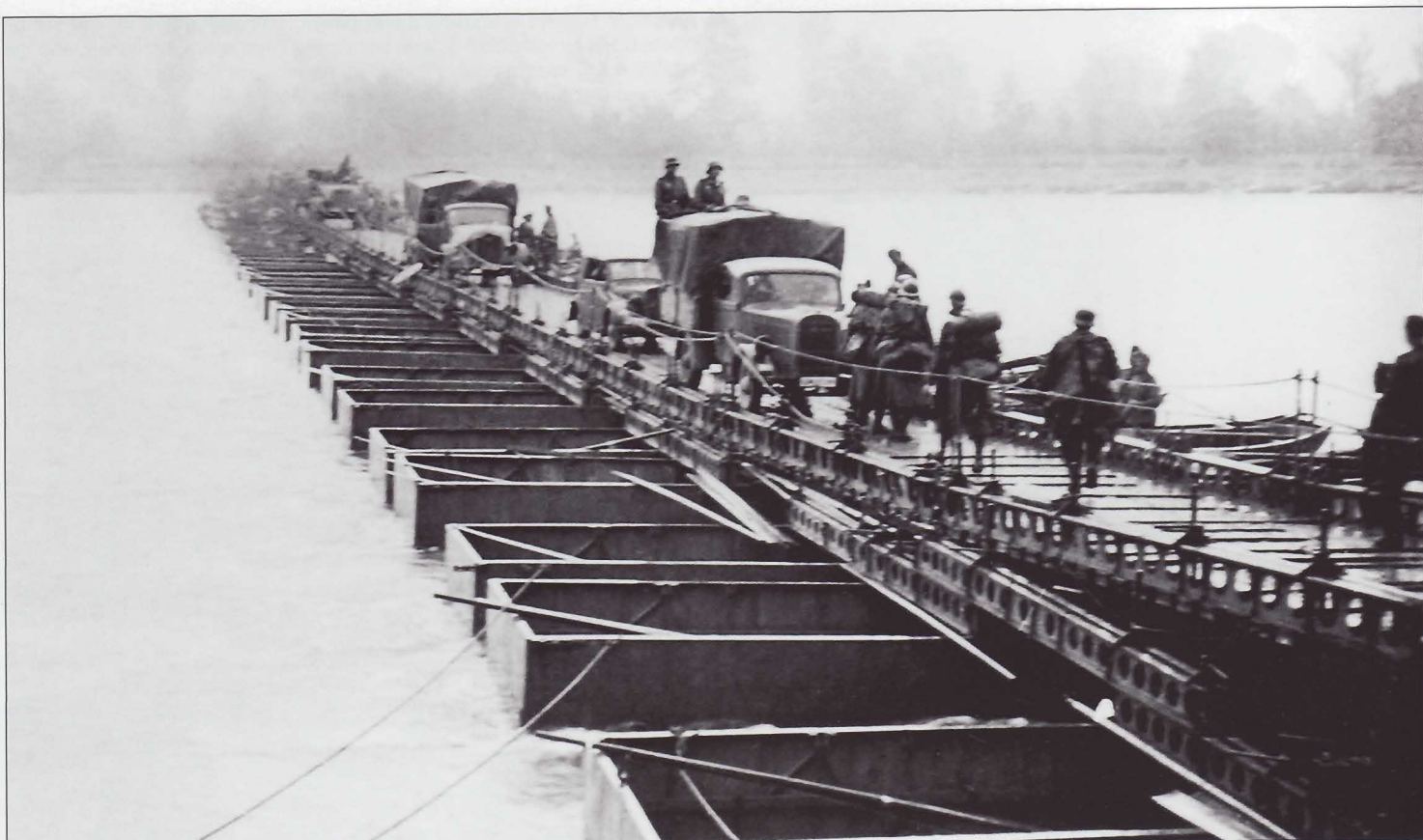
A column passes over a heavy pontoon bridge (Brückengerät B). An infantry division was assigned a fully motorized pioneer bridge column. The pontoon boats were 50 feet (15.24 meters) in length. So many rivers had to be crossed by so many different divisions that the Germans were running out of bridging equipment.
