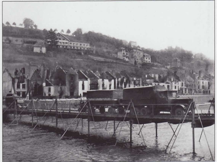
This fixed-type bridge saw little use as it required more time to erect than pontoon bridges. They often replaced pontoon bridges in rear areas so that they could be moved forward. The burnt-out buildings attest the extent of French resistance in this area. A Bussing-NAG medium cargo truck towing a 5-ton E5 standard trailer crosses the bridge.
