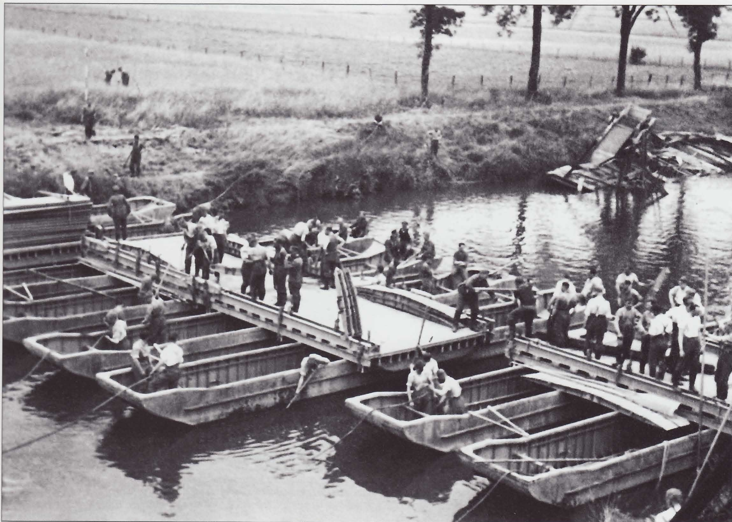
A bridge section is floated into position on two 50-foot pontoon boats. Once the bridging equipment was at the crossing site a bridge could be erected in a surprisingly short time. Note that on the far shore the pioneers preparing the approach ramp to the bridge. Finding a site with suitable egress and exit routes was the main factor in selecting a bridging site.
