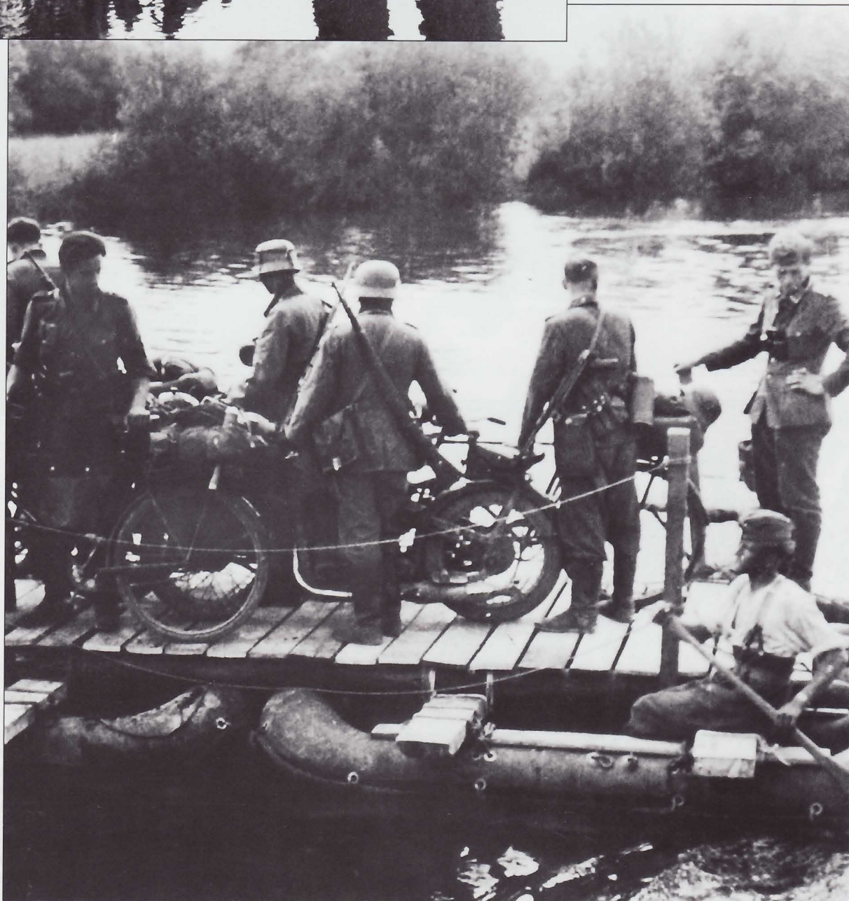
A motorcycle unit crosses a river aboard a ferry made from three-meter pneumatic boats, normally used to transport three men. These boats could also be used as pontoons for footbridges.
