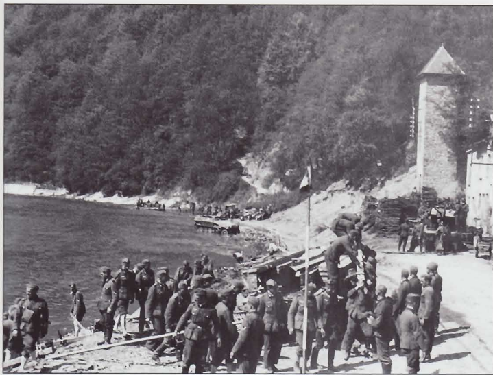
Pioneer bridge construction troops erect a fixed-type bridge over a swiftly flowing river. This type of bridge was better suited in swift, shallow rivers than pontoon bridges. It can be seen that the water level is sufficiently low and the gravel bottom solid enough for trucks to ford the river. A bridge is needed though as constant traffic would soon churn up the bottom making it impassable. The water level could rise after any rains.
