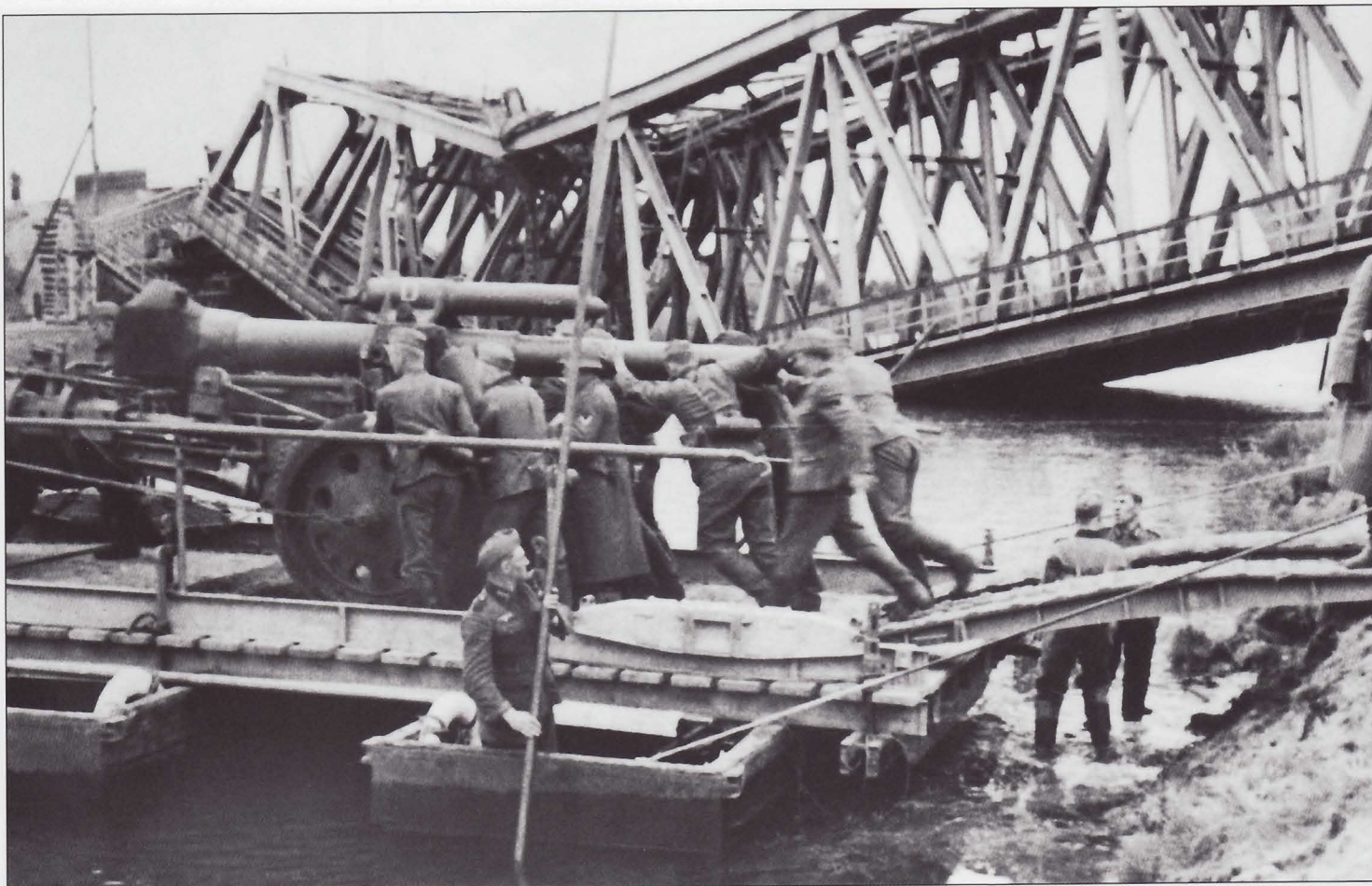
Whenever a bridge had been downed German pioneers would erect a pontoon bridge or establish a ferry-crossing site. Here three light bridge (Brückengerät C) pontoon boats have been configured into a ferry. Three pontoon boats could carry 5.9 tons and two 4.5 tons. Four-meter aluminum light assault bridge sections span the gap between shore and the ferry. The 15cm sFH18 heavy field howitzer has a "D" painted on the recoil cylinder. Each howitzer in a battery was designated by a phonetic alphabet letter: Anton, Bertha, Cäsar, and Dora.
