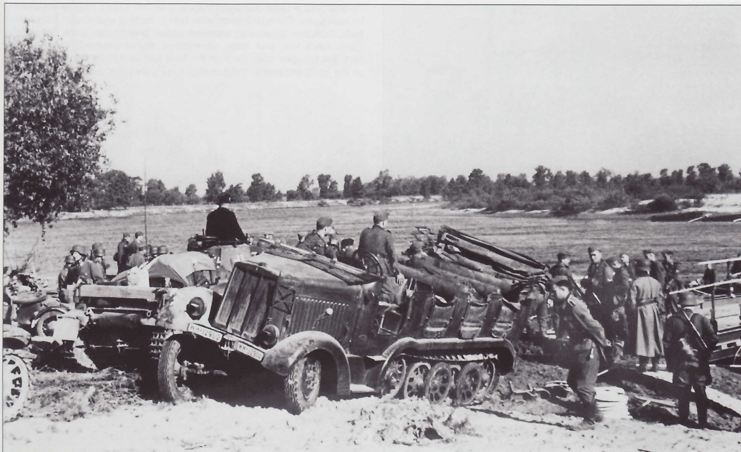
This 8-ton SdKfz 7 medium halftrack has just cross a pontoon bridge. This vehicle was normally used as a prime-mover for 15cm field howitzers, 10cm guns, and 8.8cm Flak guns. The canvas cover has been incompletely folded down.
