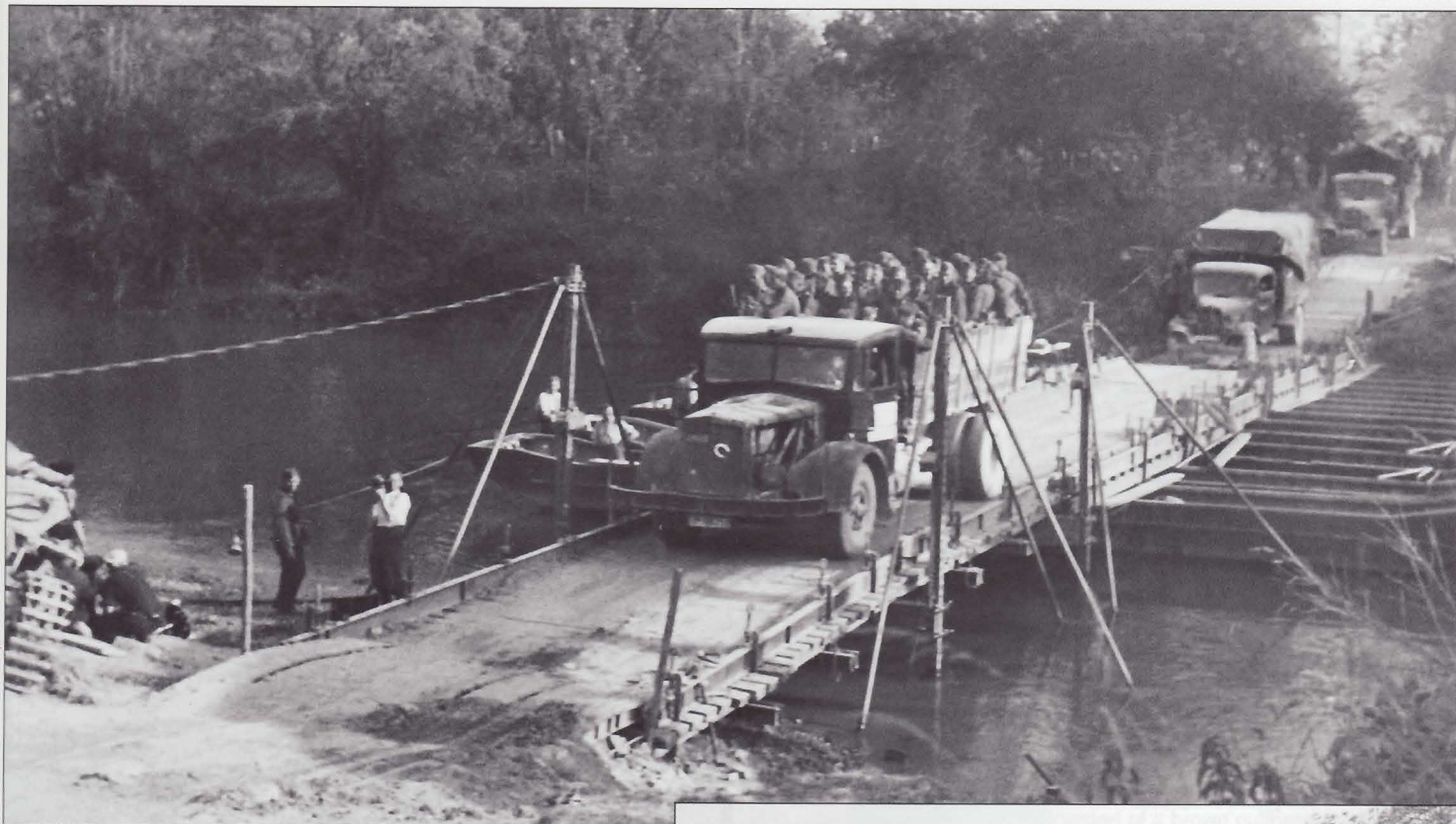
A combination fixed-type and pontoon bridge. This combination was employed when the bottom was too shallow to float pontoon boats. It is difficult to identify specific types of trucks as there were so many different makes and models employed to include commercial models and vehicles commandeered or purchased before the war from Czechoslovakia, Austria, Poland, etc. Truck "45" passing through this burning town was built by Ford Werke of Cologne.
