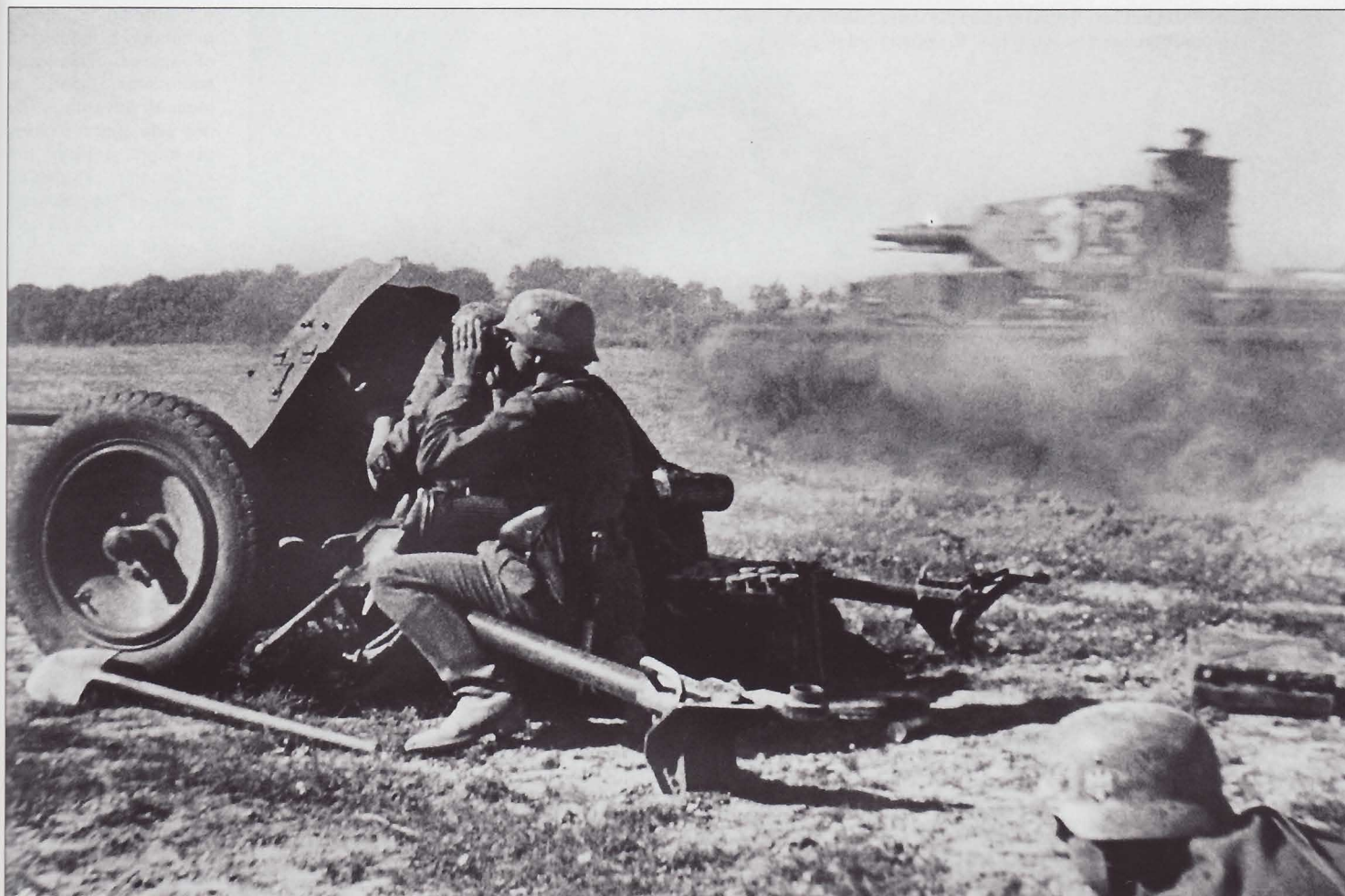
A 3.7cm PaK 35/36 antitank gun provides covering fire as a PzKpfw IV advances toward a treeline. The PzKpfw IV was at the time considered to be an infantry support tank. It was the heaviest tank in the German inventory and few in number, less than 300, but it was not thought of as a tank-fighter. It had a short 7.5cm KwK 37 L/24 gun intended for knocking out field fortifications. The tanks were not to advance no more than 100 meters ahead of the infantry. They were also to act as artillery forward observers to direct artillery fire in support of the infantry when other observers were unavailable. The short bar below the barrel served to deflect the radio antenna with the turret traversed.
