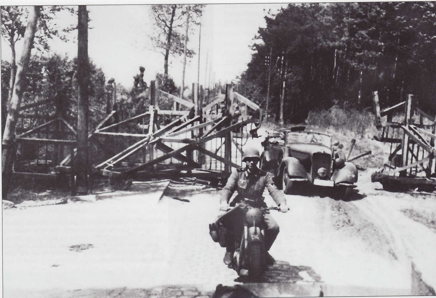
A column passes through an antitank barrier built of Belgium semi-portable obstacles known as "C" elements. There were later used as underwater obstacles on the Atlantic Wall and known to the Allies as "Belgium gates." The twisted damage suffered by the "C" elements on either side of the staff car indicates they were blown open by demolition charges.
