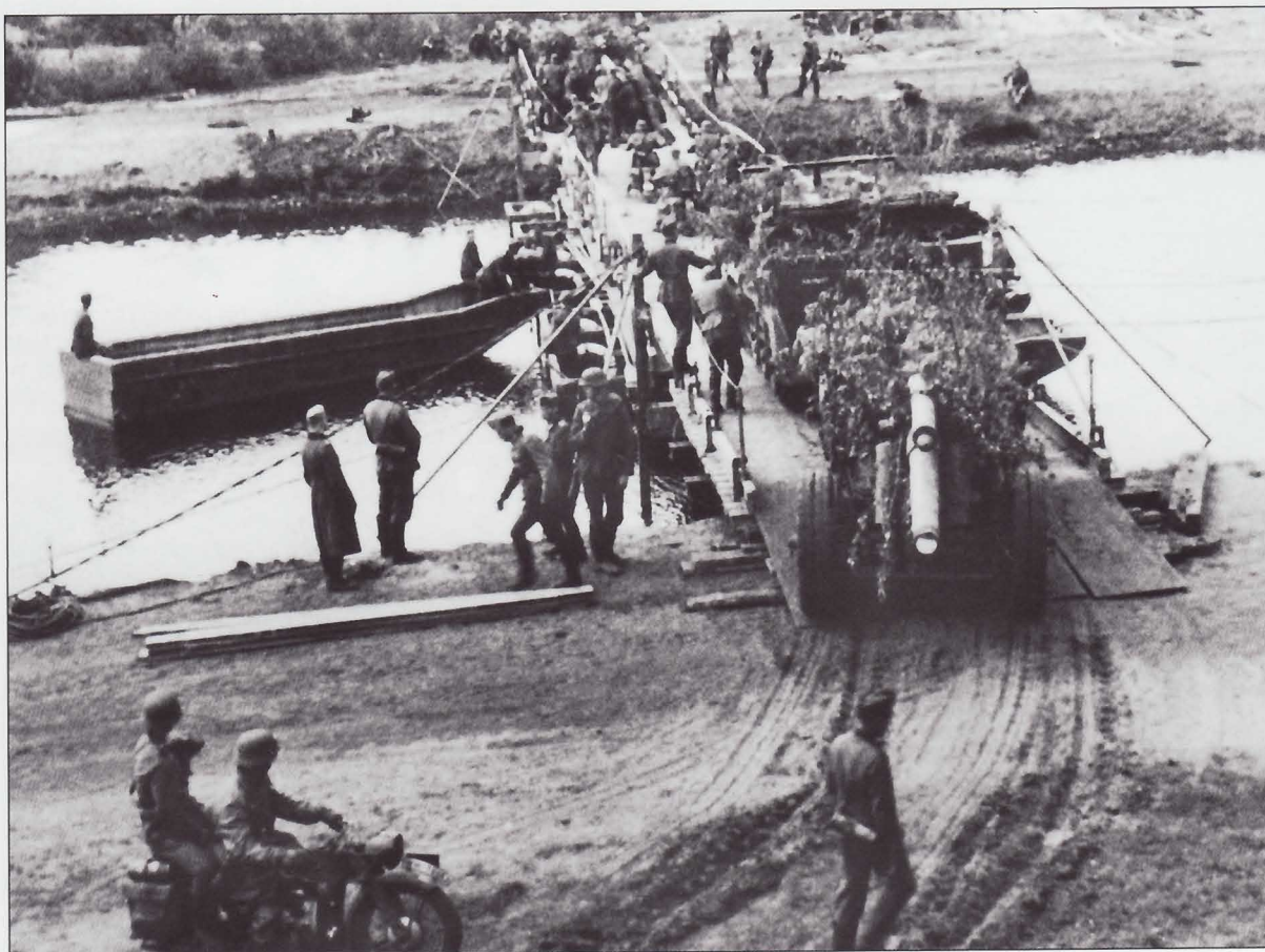
Whenever a bridge had been downed German pioneers would erect a pontoon bridge or establish a ferry-crossing site. Here three light bridge (Brückengerät C) pontoon boats have been configured into a ferry. Three pontoon boats could carry 5.9 tons and two 4.5 tons. Four-meter aluminum light assault bridge sections span the gap between shore and the ferry. The 15cm sFH18 heavy field howitzer has a "D" painted on the recoil cylinder. Each howitzer in a battery was designated by a phonetic alphabet letter: Anton, Bertha, Cäsar, and Dora.
